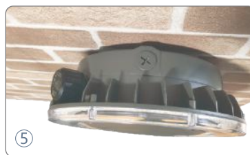
5. Slide the fixture one the plate.
