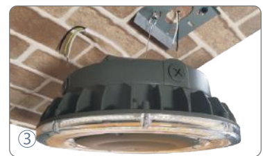
3. Hanging the fixture on one of the installation screws.
