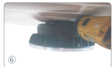
6. Tighten the two screws to lock the fixture on the plate.
